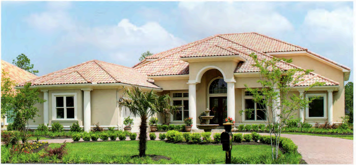
The professional landscaping and brick-paved driveway add tremendous curb appeal to this custom home in Plantation Lakes, SC. A hard-coat stucco system was used on the exterior and Buttercup Blend Spanish "S" concrete tiles for the roof.
